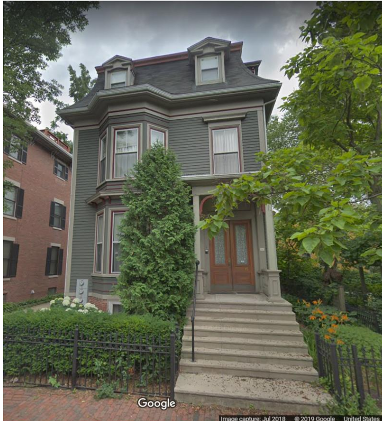
Figure 11. This is the building at 310 Harvard St in Cambridge hand restored by the Bolognas. Their renters took advantage of them, didn't pay rent for five years, couldn't be evicted and illegally sublet at market rent. The Bolognas were fined $64,000 by the rent board, had another $30,000 in attorney fees, and ultimately lost the house to bankruptcy. They are not landlords anymore. in https://goo.gl/maps/Kv3j2qrnFxFMFA5U9
